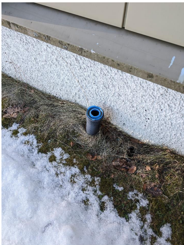
Figur 6 Antatt stakerør for drenering.
